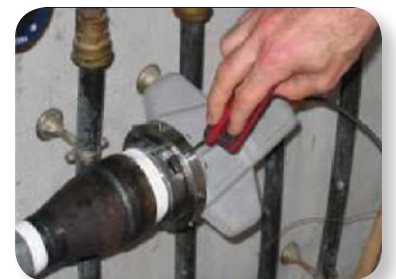
Figure 2: WT 230L sound emitter connected to a pipeline under test.*
